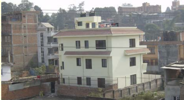
View of LBU2 from LBU1's roof
